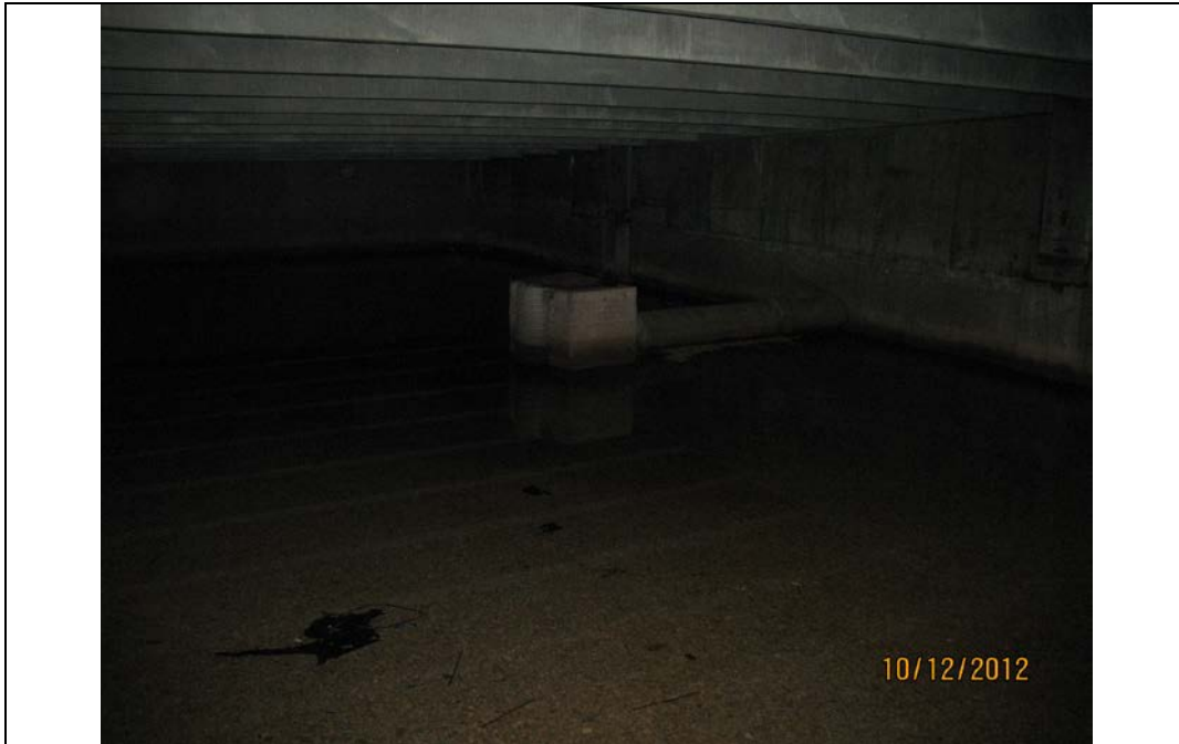
Photo No. 53. Sample location 4 th Ave. Garage, view to the NW from entrance of vault
