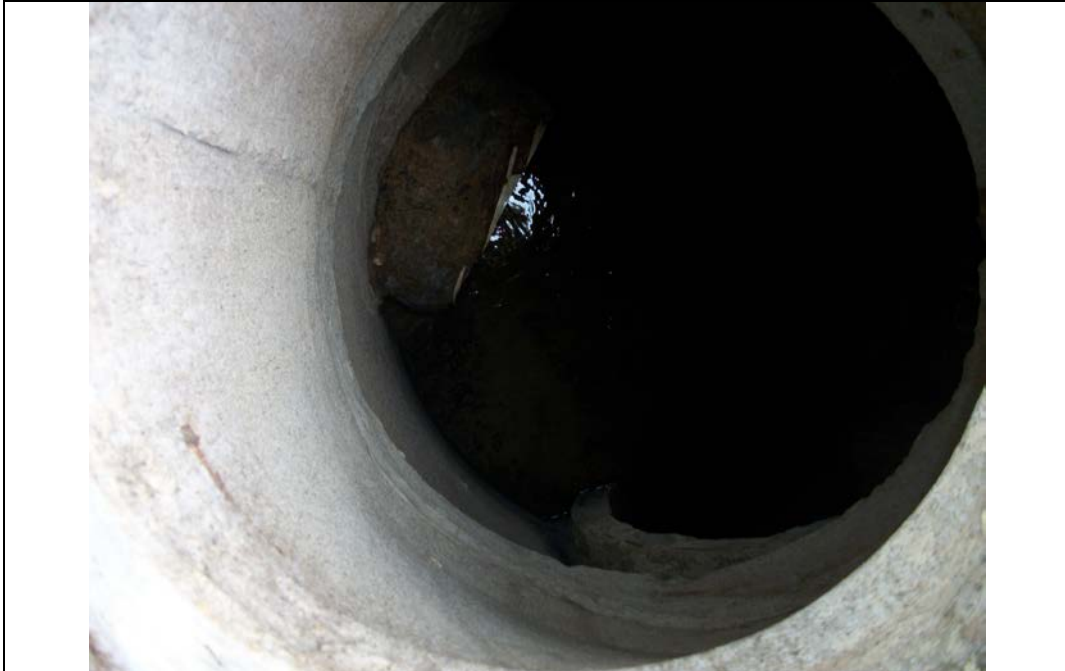
Photo No. 58. Sample location CP, view into manhole, N is up
