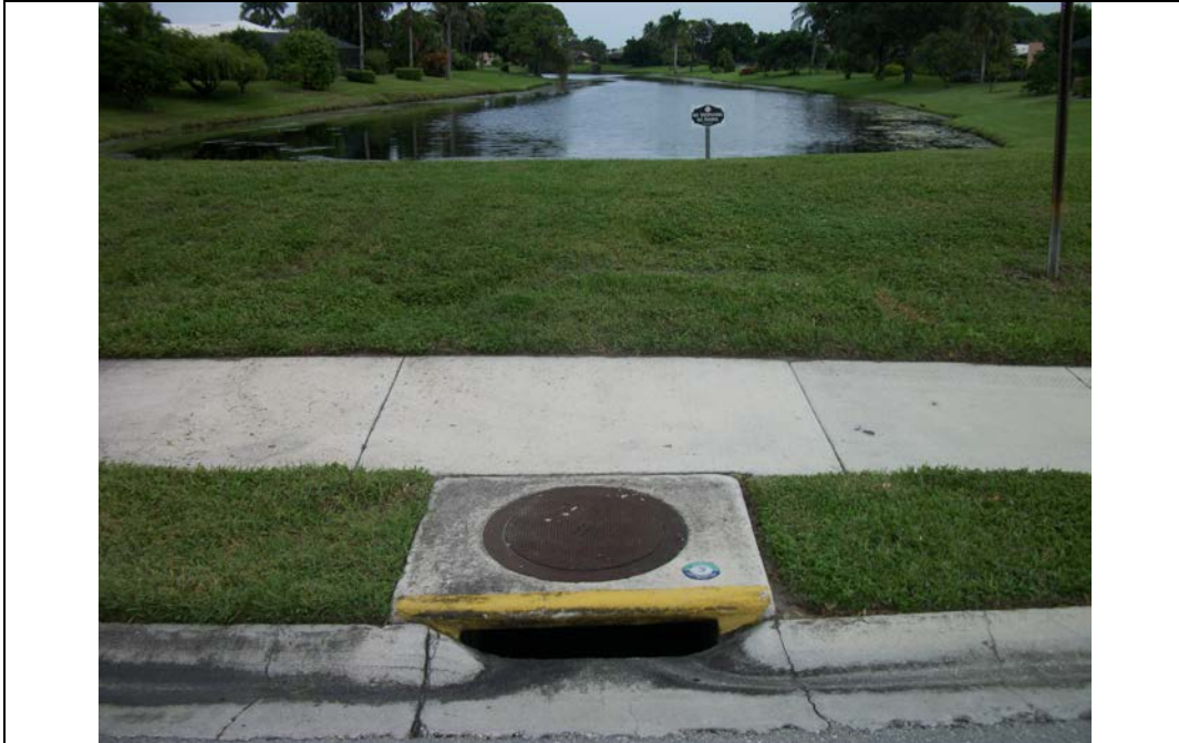
Photo No. 62. Sample location 1A3, view to the S
