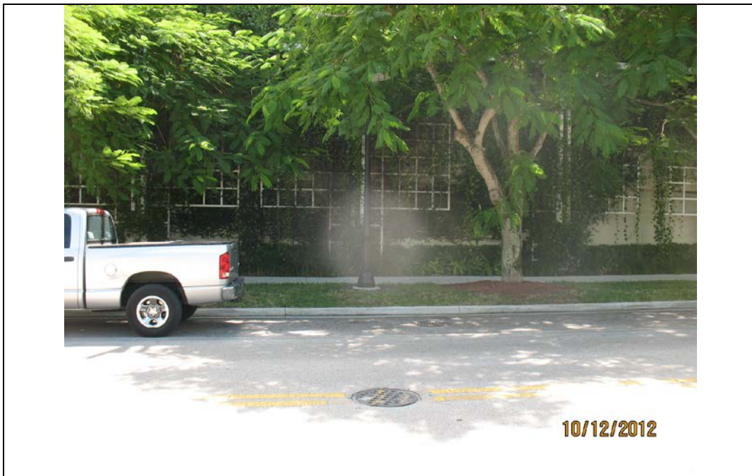
Photo No. 54. View of manhole street-side of sample location 4 th Ave. Garage, view to the S
