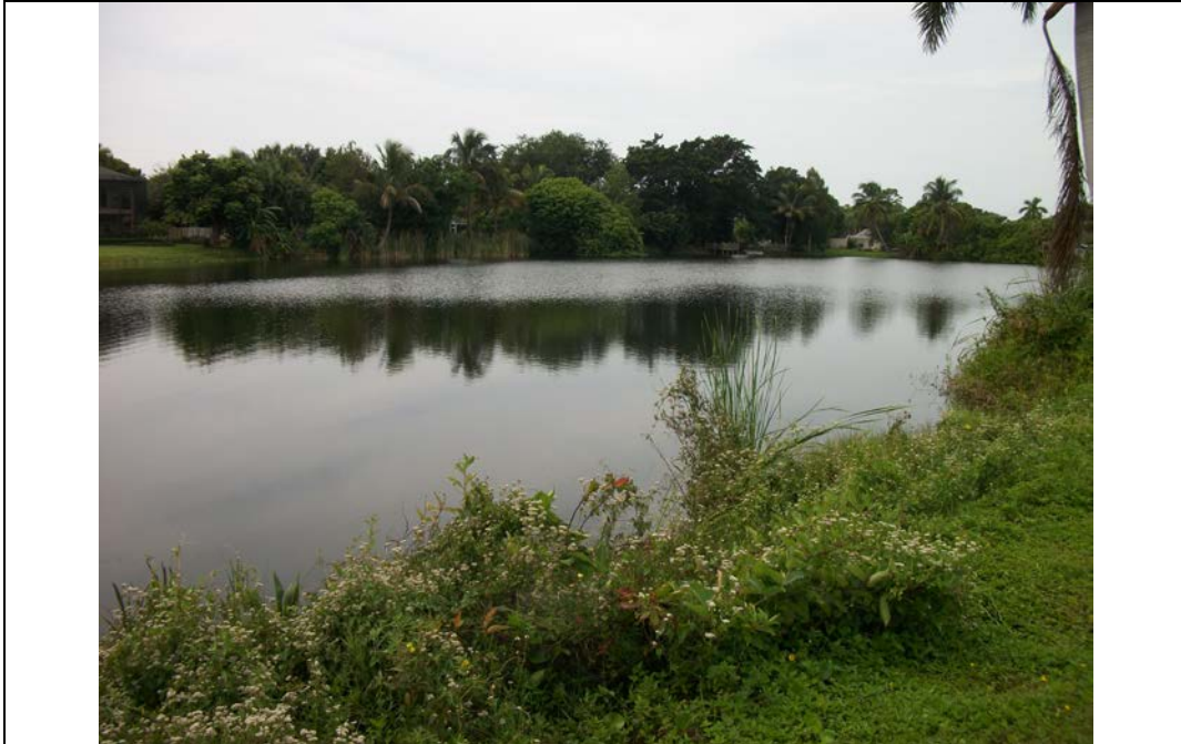
Photo No. 37. Lake 19, view from outfall to the SW
