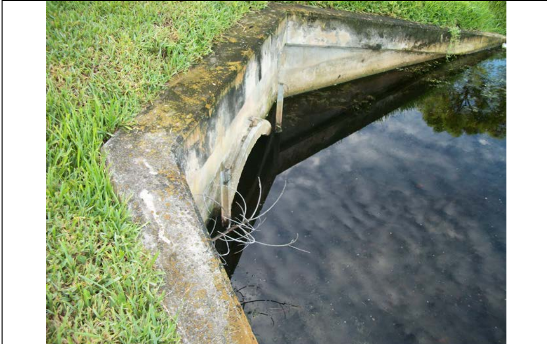
Photo No. 47. Sample location 1A, view to the S
