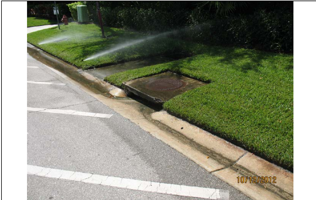
Photo No. 57. Sample location GD, note sprinklers were not on at time of sample collection, sample taken from grate that discharges into curb inlet
